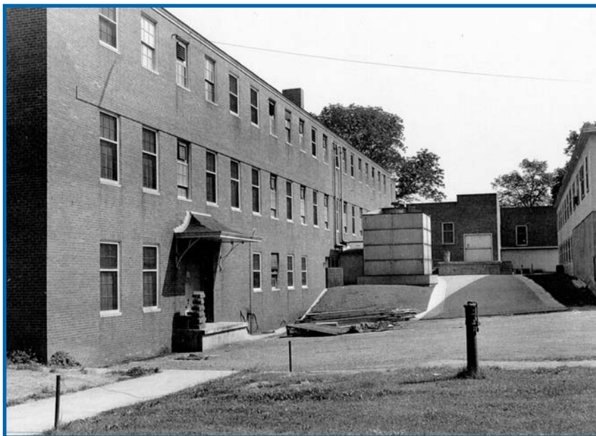
U.S. Navy Communications Annex, Building 4
