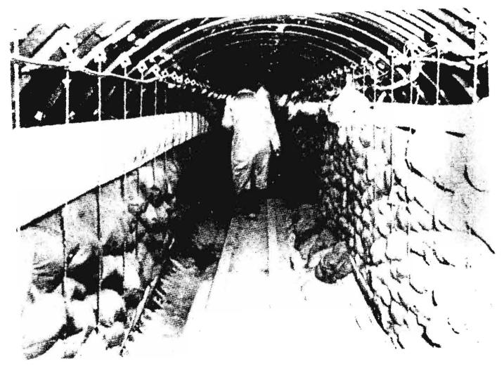
A Soviet photograph taken from just beyond the chamber where the landline taps were applied. Intercepted signals were relayed to the U.S. sector through the cables shown at the lower right corner of the passageway.
