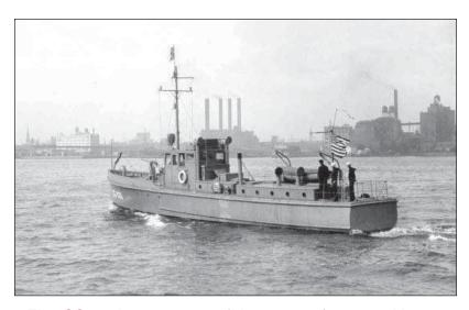
The *CG-100* in 1928, one of the 203 75-foot patrol boats built for Coast Guard Prohibition enforcement duties. Known as "six-bitters," they entered service between 1924 and 1925. With a top speed of 15 knots, they were slower than most rumrunners but well built for off-shore operations. (Photo by Joseph N. Pearce, U.S. Coast Guard)
