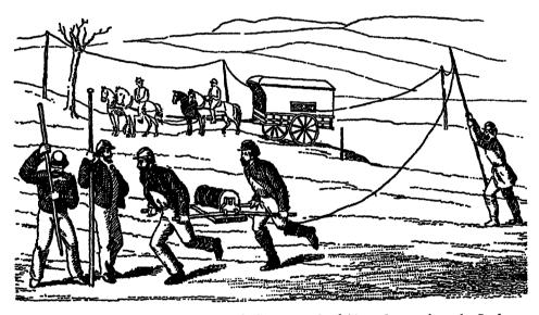
A drawing from Myer's Manual of Signals illustrating the field, or flying, telegraph. It shows the wagon with batteries and instruments. The wire (in this case presumably bare copper, since it is being strung on insulators on poles) is being run out from a reel carried by two men. The linesmen are using a crowbar to open holes to receive the lance poles. Myer estimated that 2½ miles of such wire line could be put up in an hour.
