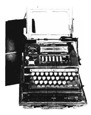
Menzer Device SG-41. A successful encipherment system, but of limited use due to its heavy weight.
