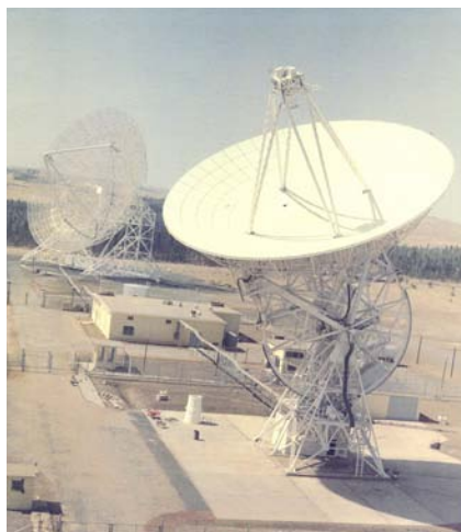
Now-closed STONEHOUSE deep space TELINT facility
