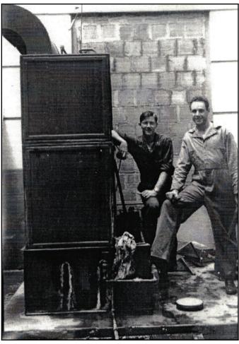
Fig. 12. SIGSALY's air conditioning system<sup>23</sup>
